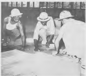
THOUSANDS OF square feet of coral and grey rubber tiles had to be laid. MILES DI pia cuadrá di azulejo color coral y shinishi mester a worde poni.
